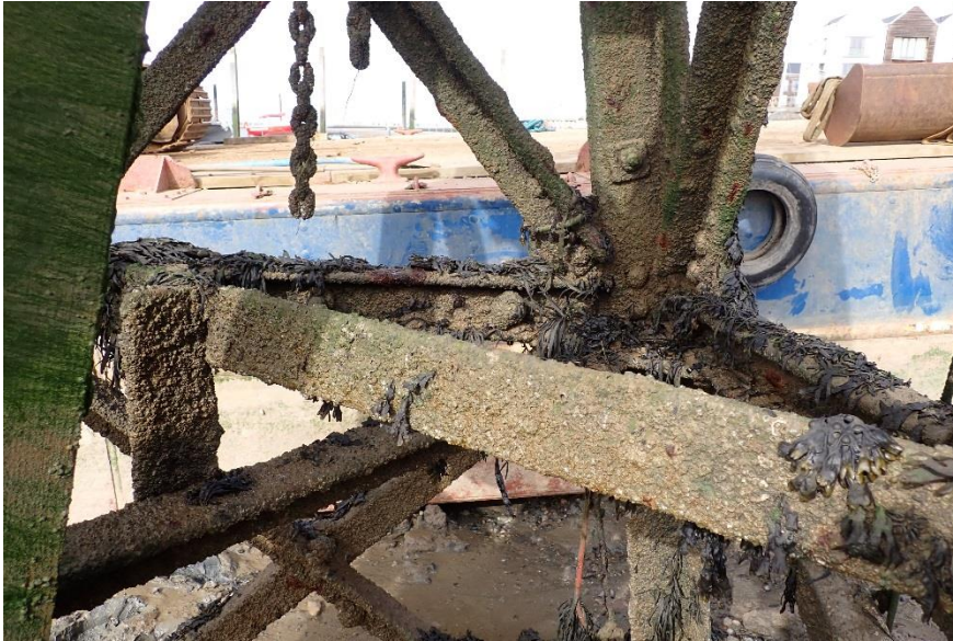
Fig 19 – Dolphin 3 at high tide mark interior bracing
