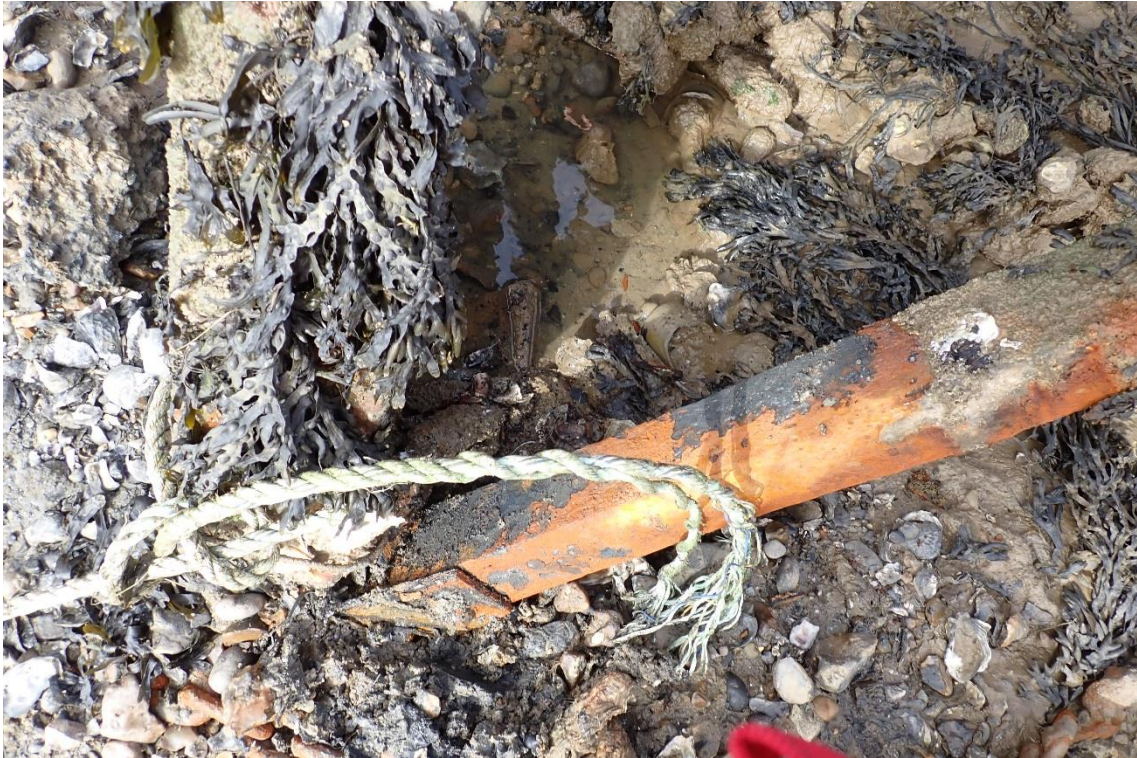
Fig 25 - Dolphin 3 at mud line following removal of marine growth
