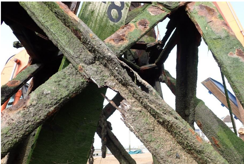
Fig 20 – Dolphin 3 typical condition of members at high tide line
