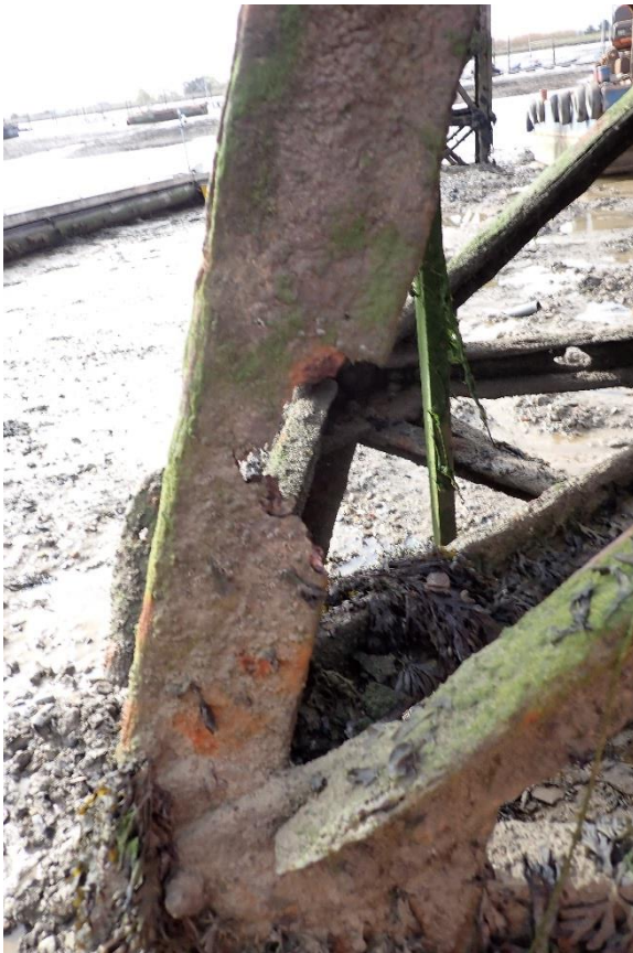
Fig 5 & 6 – Results of hammer testing on Dolphin 1
